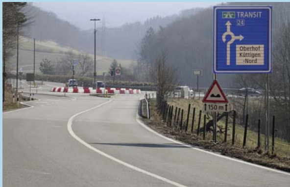
NK107 Neue Staffeleggstrasse
